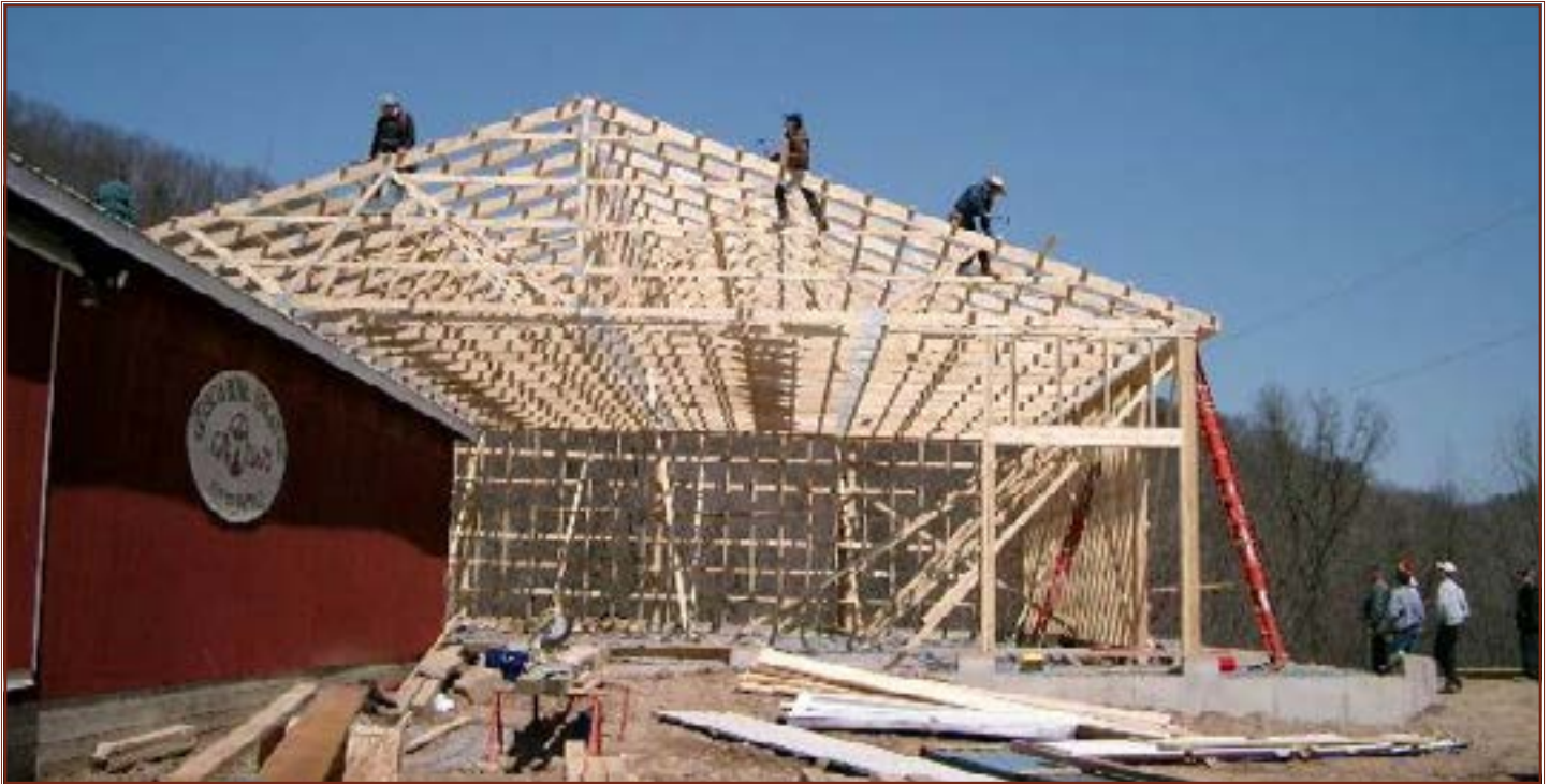
Construction of 2004 addition.
